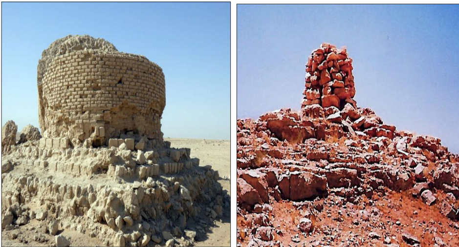
Fig :3.4 .Photographs of the construction of the Almushraf in Zubaydah Trail) the one on the left( consisting of an old cylindrical brick building) the one on the right (of Almushraf built in the form of a stone cylindrical structure) The Desert Team Trail 1) July.(2022 ,4)
