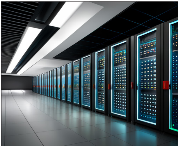
Figure 8 Predictive platforms and central control
