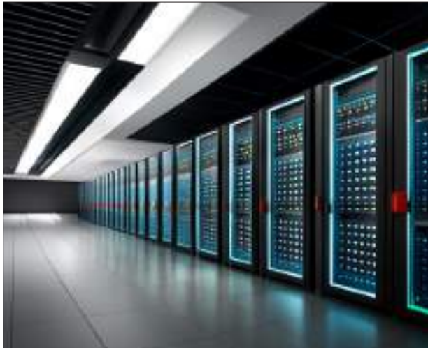
Figure 8 Predictive platforms and central control
